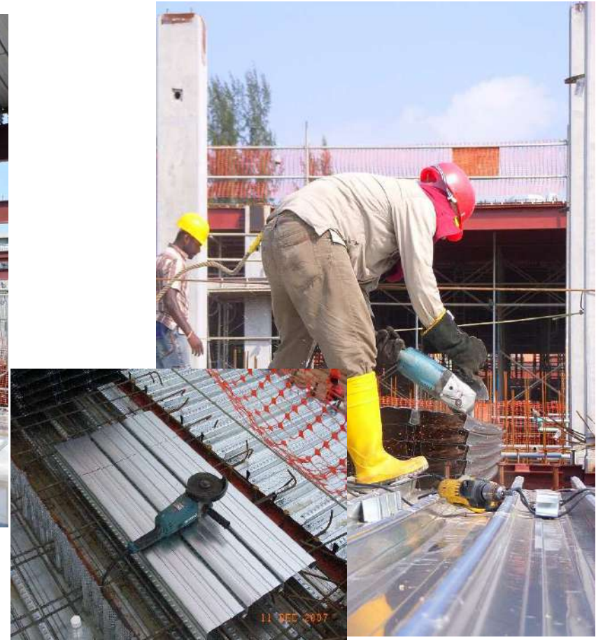
BONDEK II can be cut on site using simple tools
