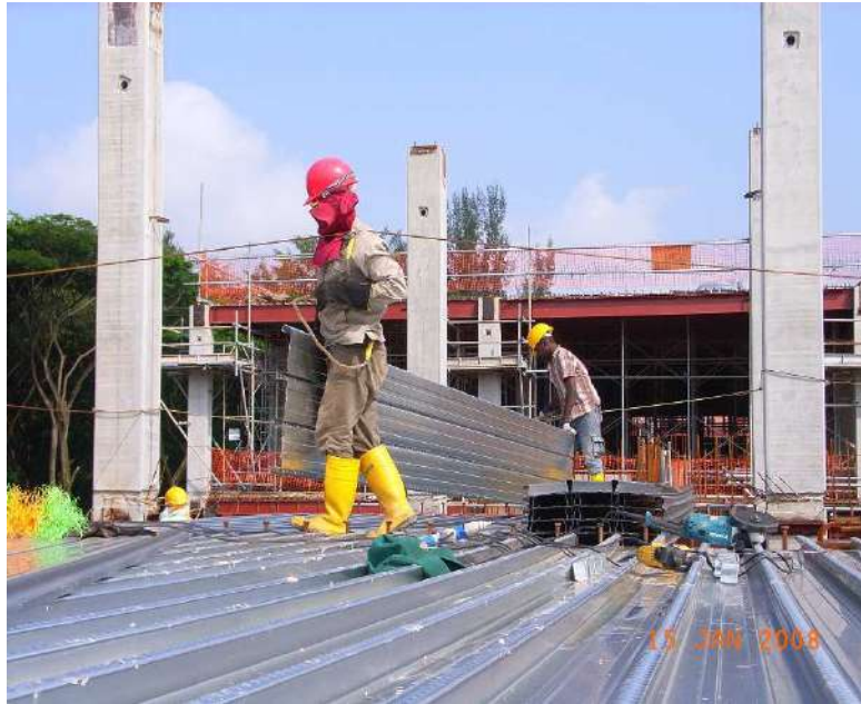
Laying is done with no machine aid
