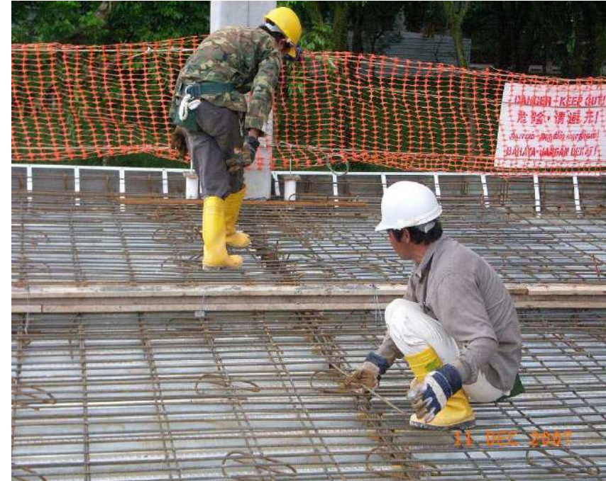
Lay the reinforcement bars
