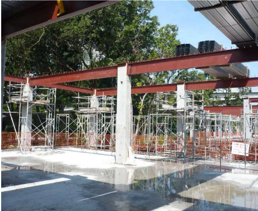
BONDEK II bundles hoisted onto steel frames
