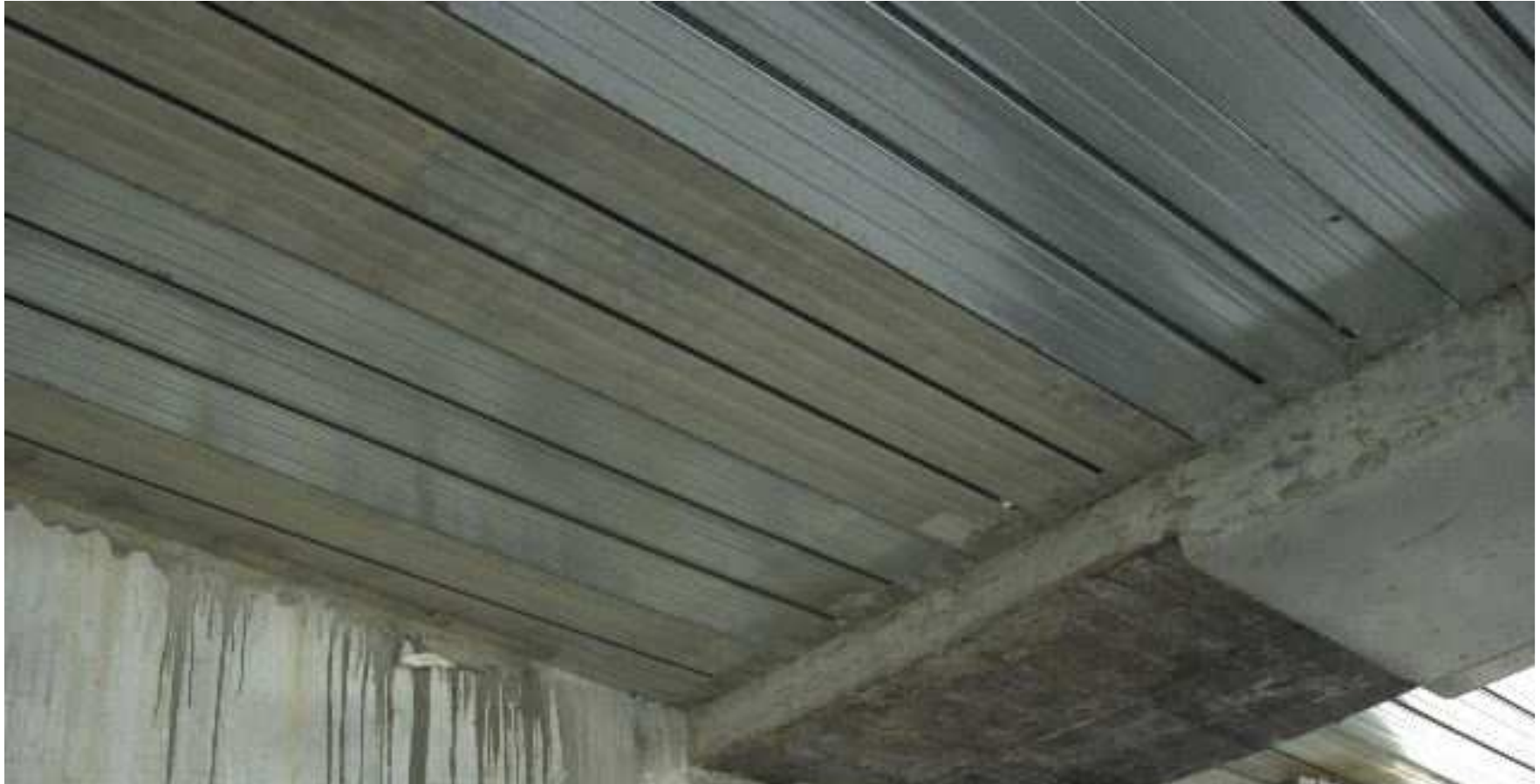
LYSAGHT BONDEK II - BAHRAIN FINANCIAL HARBOUR (UNDERSIDE OF LYSAGHT BONDEK II)
