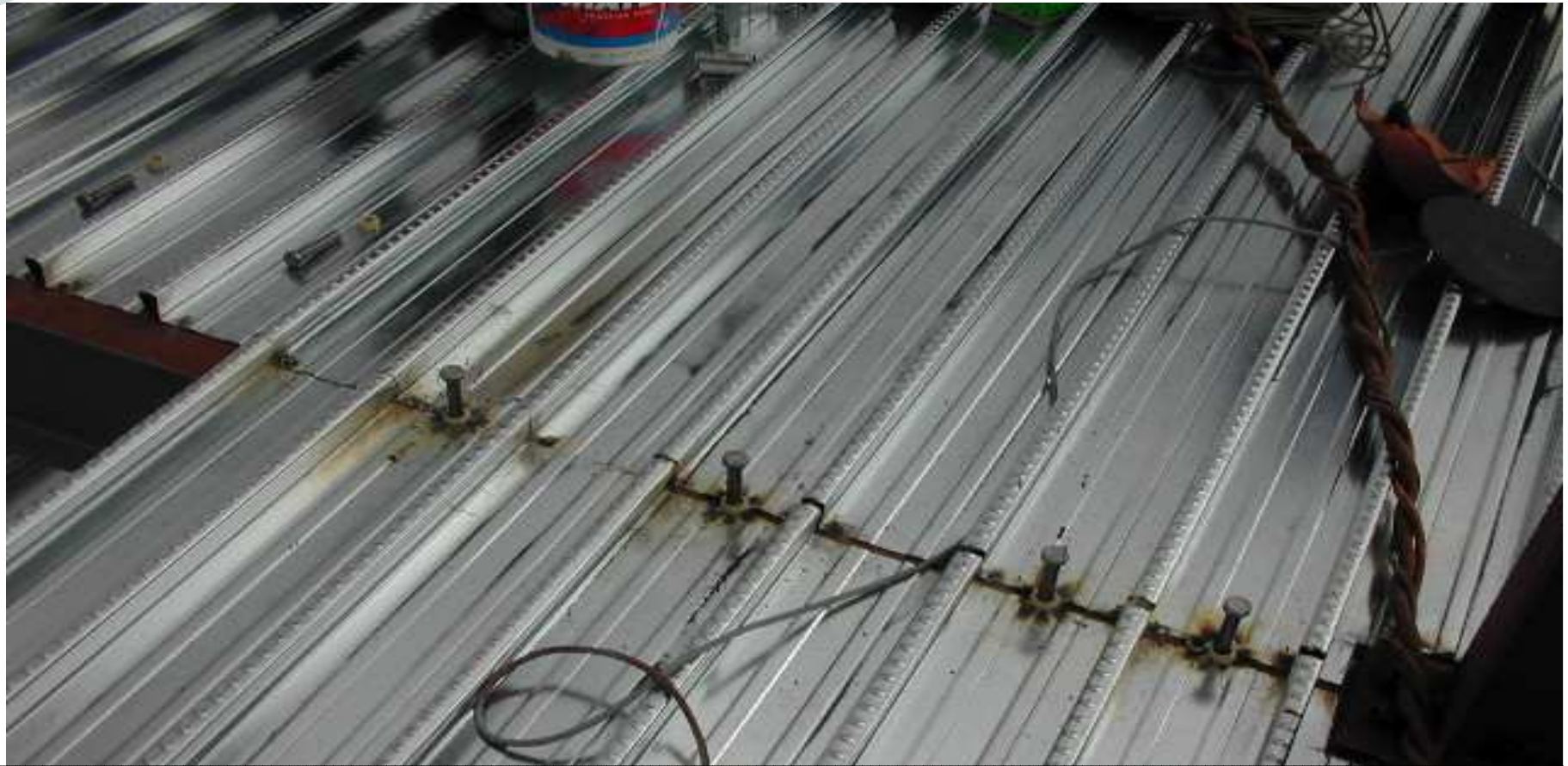
SUBANG AIRPORT - INSTALLATION OF SHEAR STUDS
