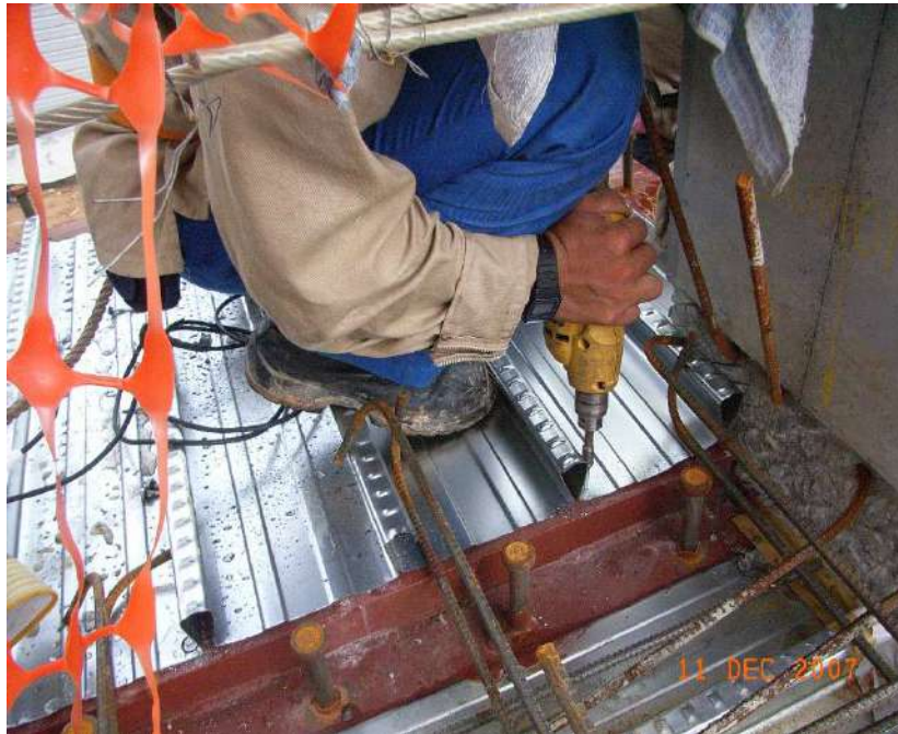
Secure BONDEK II to steel beams
