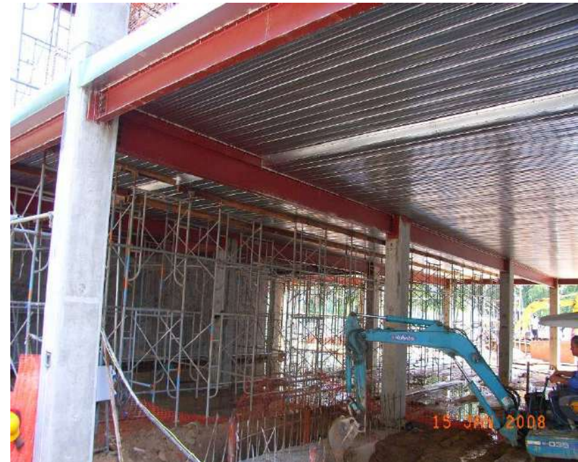
Provide necessary Propping
